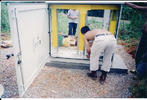
Inside Installation of Storage Module and Cable Management
