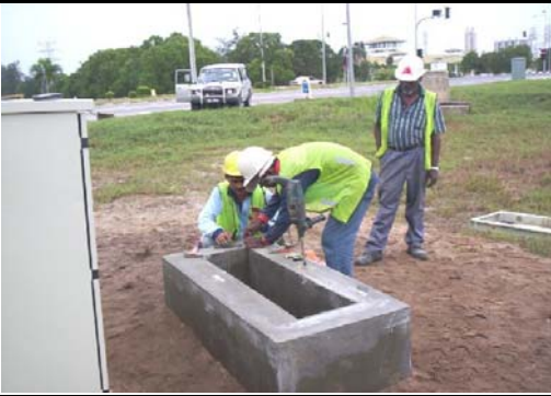
After concrete hardern (usually 2-3 days) formwork shall be strip off
