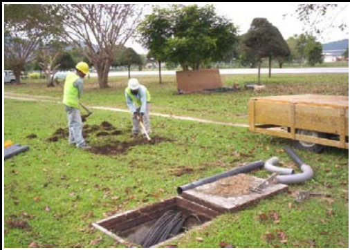
Preparation of Excavation
