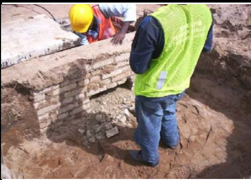
Erection of brick wall for manhole
