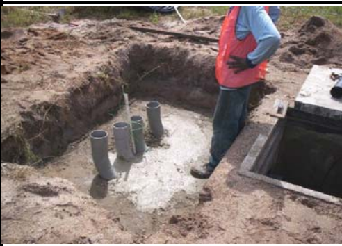
Completing Duct Work
