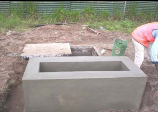
After concrete hardern (usually 2-3 days) formwork shall be strip off
