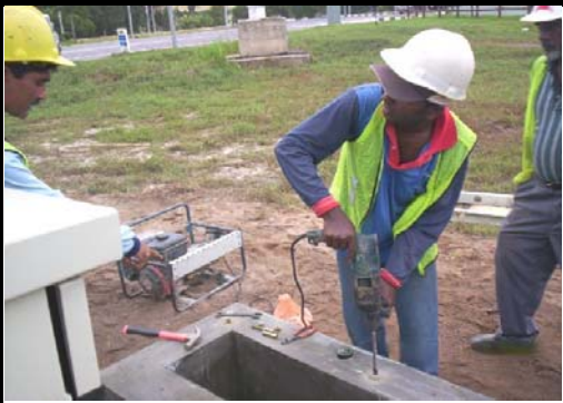
Installation of raw plug for mounting the FEDB
