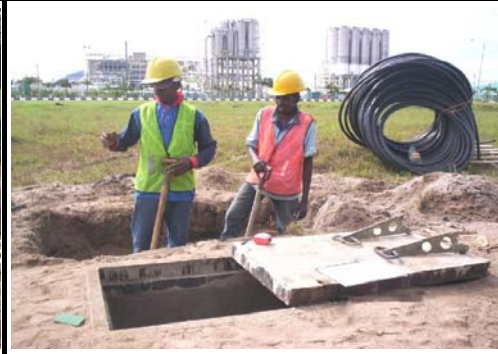
Excavation preparation for plinth and manhole
