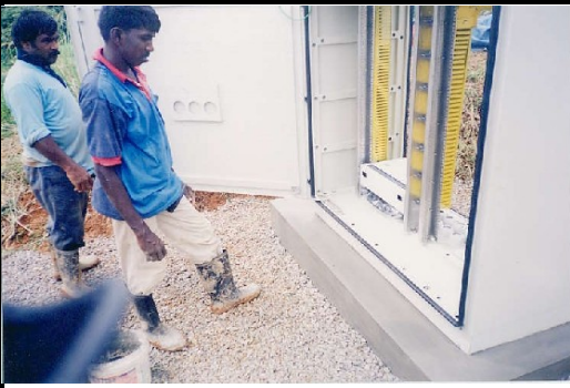
Inside Installation of Storage Module and Cable Management
