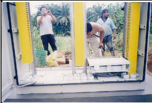
Inside Installation of Storage Module and Cable Management
