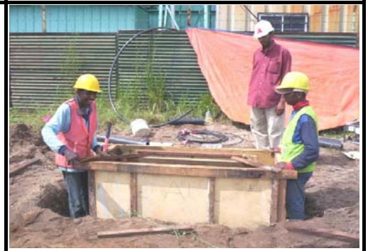
Service trenching formwork placed in position and continue next level of concreting
