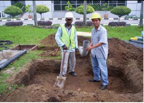
Pit are diggup to allow long bend lead into manhole
