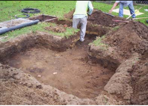
Excavation (pit) ready for Plinth
