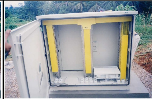
Inside Installation of Storage Module and Cable Management
