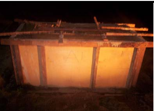
Service trenching formwork placed in position and continue next level of concreting
