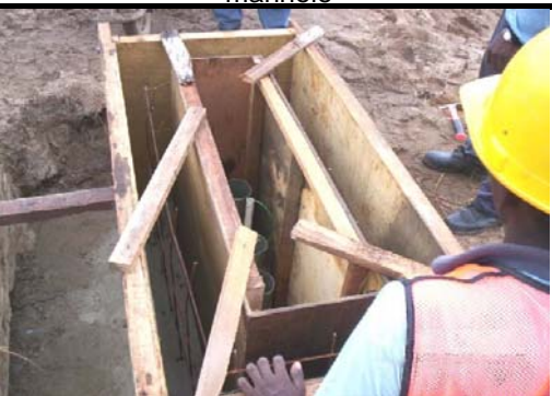
Service trenching formwork placed in position and continue next level of concreting
