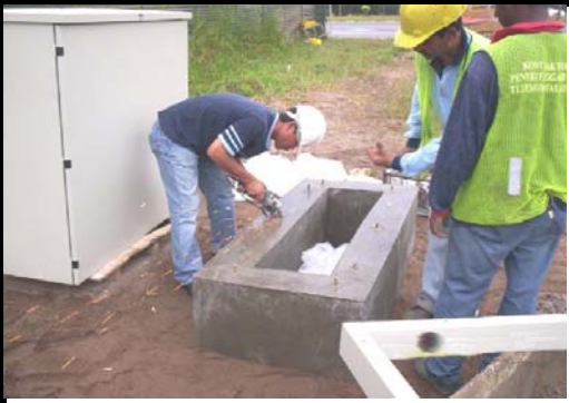
Installation of raw plug for mounting the FEDB
