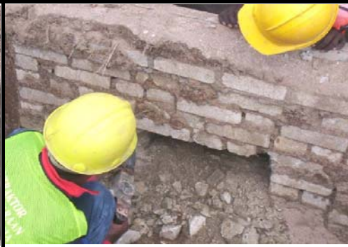
Erection of brick wall for manhole
