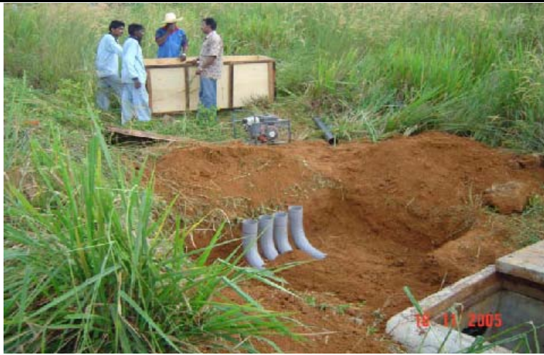
Ducting for manhole
