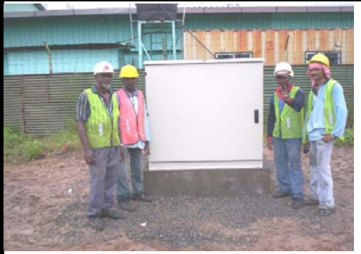
Completed FEDB and Ready for Service
