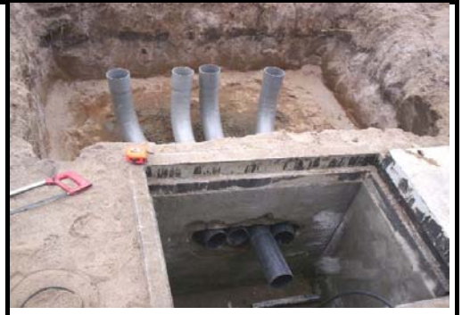
Ducting for manhole
