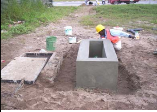
After concrete hardern (usually 2-3 days) formwork shall be strip off
