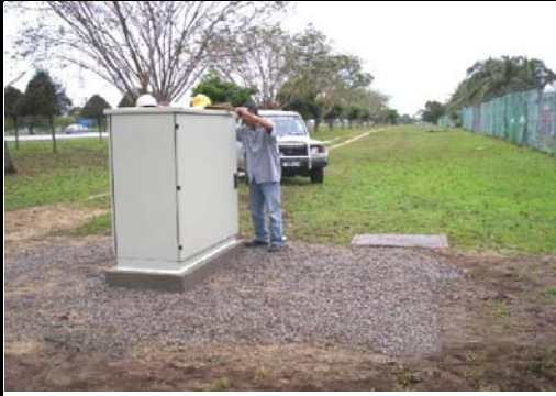
Calibrating FEDB surface levels
