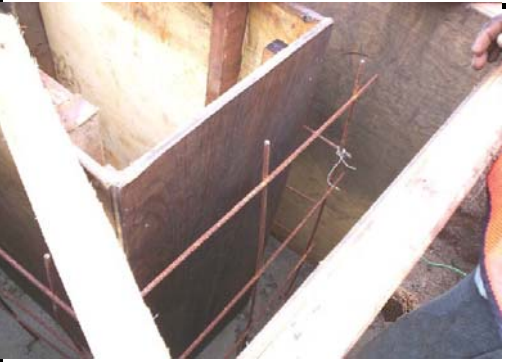
Service trenching formwork placed in position and continue next level of concreting
